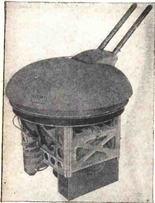
Electronically-controlled turret of a B-29.
